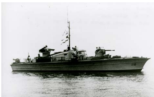
MGB 116 - British Power Boats 71ft 6in MGB. Fitted with power operated 2pdr forward, twin 20mm Oerlikon aft and twin .303 abreast of bridge.
